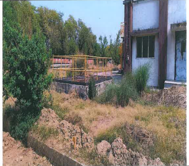
4- GTG-CPP Substation Building
