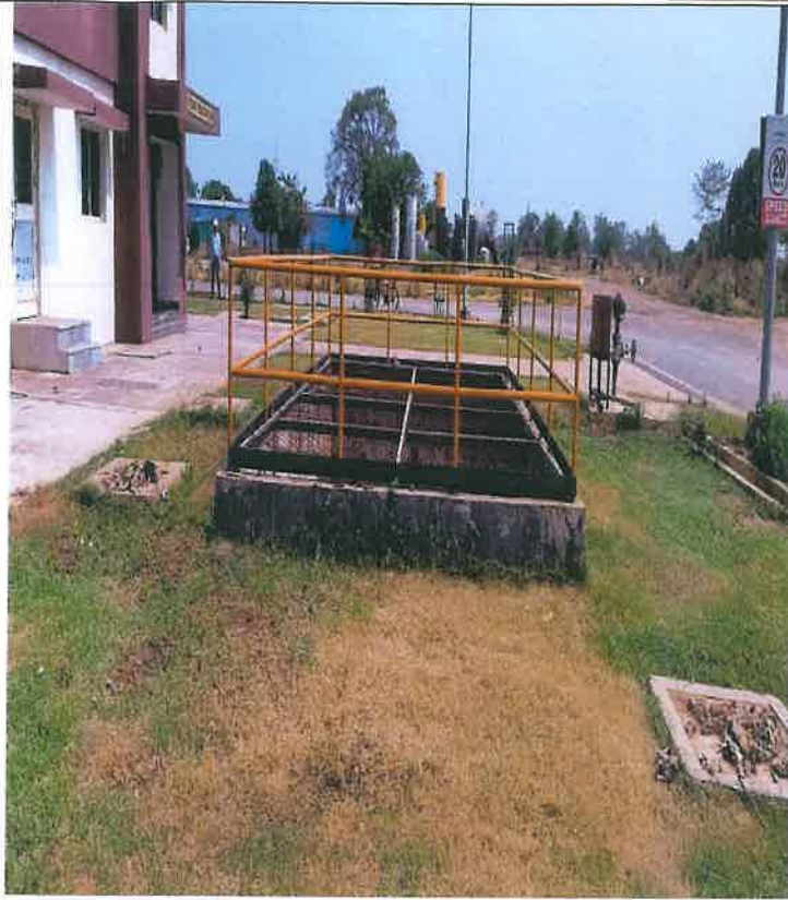
5-Ammonia Storage Tank
