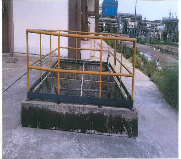
2- ACT-UCT Substation Building
